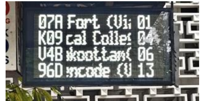
PIS Board at PMG Bus shelter
